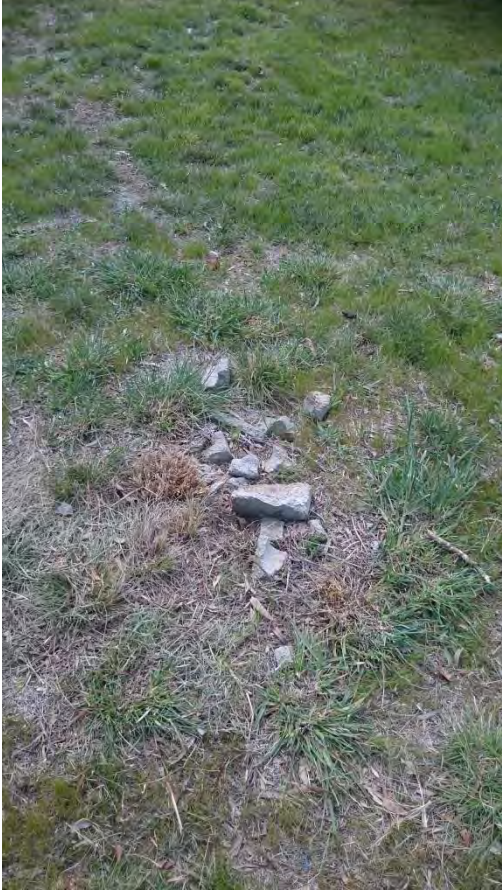
Photograph 6. Example of concrete sitting on the soil surface.
