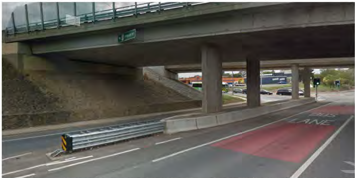
Figure 27: F-Type roadside barrier arrangement within median (Source: Google Maps)
