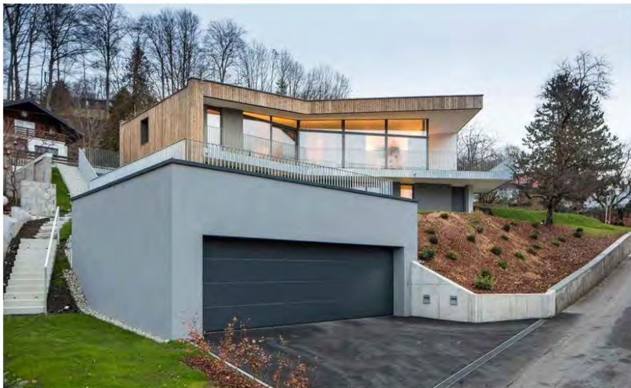
GARAGE FORWARD OF THE BUILDING LINE - REDUCED STEEPNESS OF DRIVEWAY
