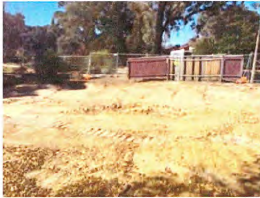
Cleared area of the demolition zone
