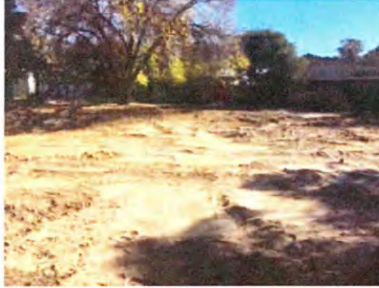
Cleared area of the demolition zone
