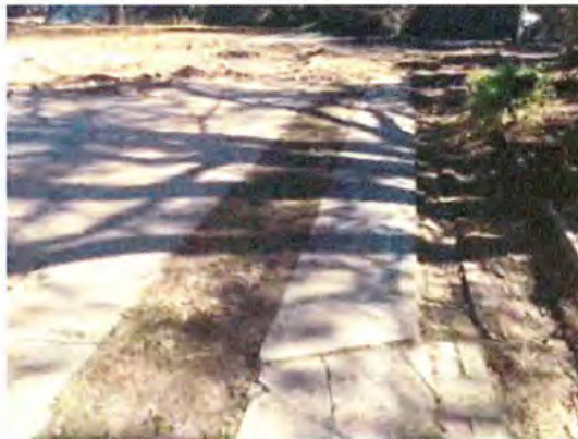
Driveway outside the demolition zone
