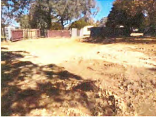
Cleared area of the demolition zone
