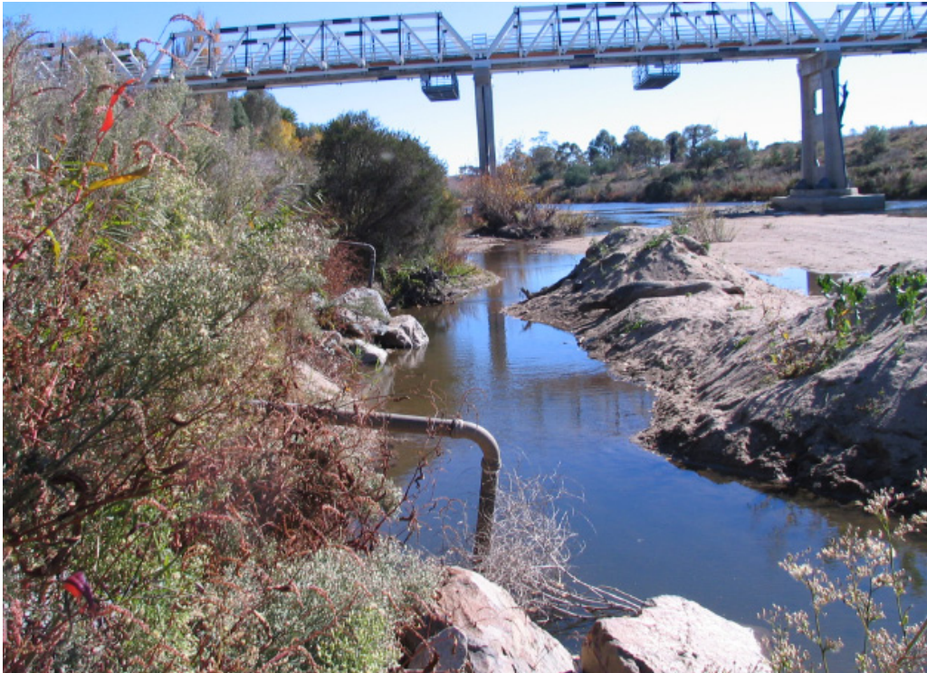
Photograph No. 16 – Pump Sheds on the bank of the Murrumbidgee River - [redacted] on the left and School system on the right – note electrical connection and exposed poly pipe and bushfire fuels
