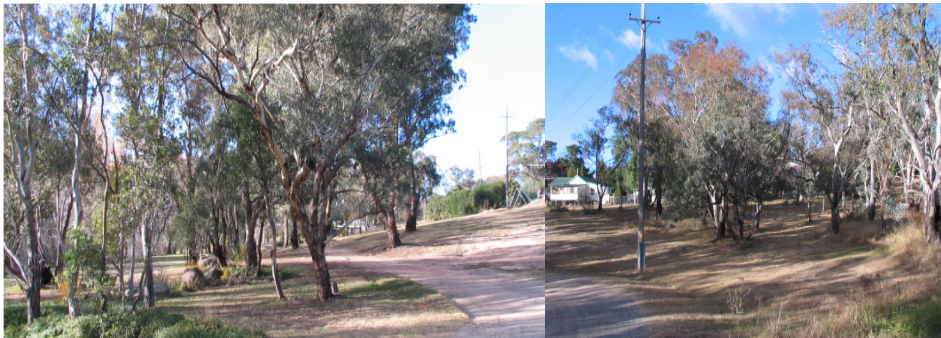
Photograph No. 3 – Looking southeast to the dwelling/s on North Street showing the managed river corridor to the northwest of the Tharwa Bridge.
