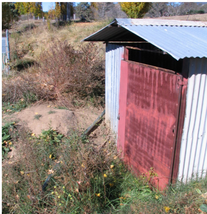
Photograph No. 17 – [REDACTED] Pump enclosure showing exposed pipe work with no protection against ember attack.
