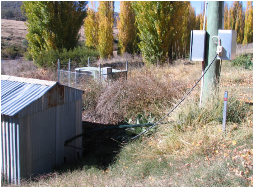
Photograph No. 16 – Pump Sheds on the bank of the Murrumbidgee River - [redacted] on the left and School system on the right – note electrical connection and exposed poly pipe and bushfire fuels
