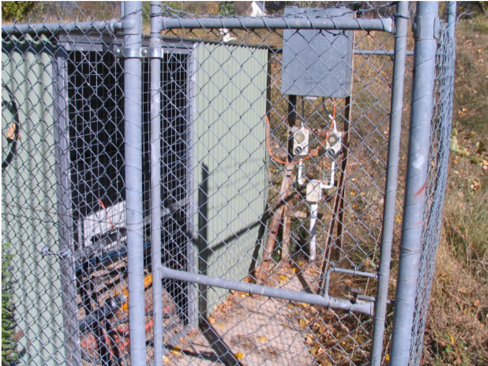
Photograph No. 17 – [REDACTED] Pump enclosure showing exposed pipe work with no protection against ember attack.
