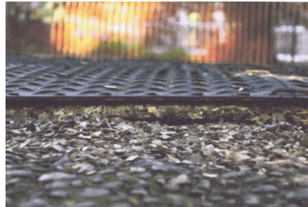
Figure 3 Ground protection (for up to 3 tonne) includes 75mm of wood chip with mats over the top.
