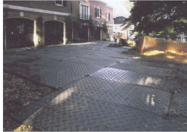
Figure 2 Example of the use of LSS for surface protection
