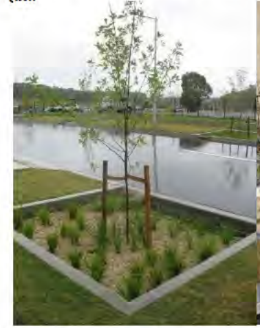
BIORETENTION STREET TREE, CRACE, ACT
