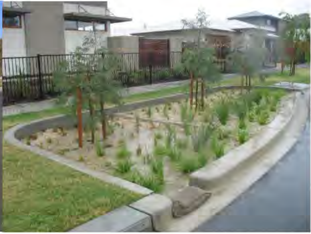
BIORETENTION RAINGARDEN IN WET WEATHER, CRACE, ACT
