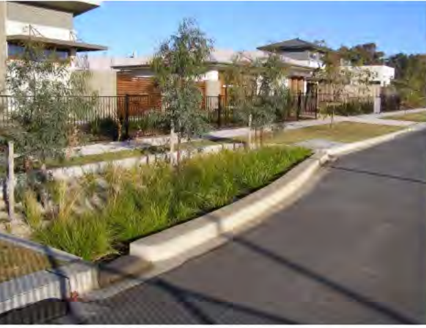
BIORETENTION RAINGARDEN, CRACE, ACT
