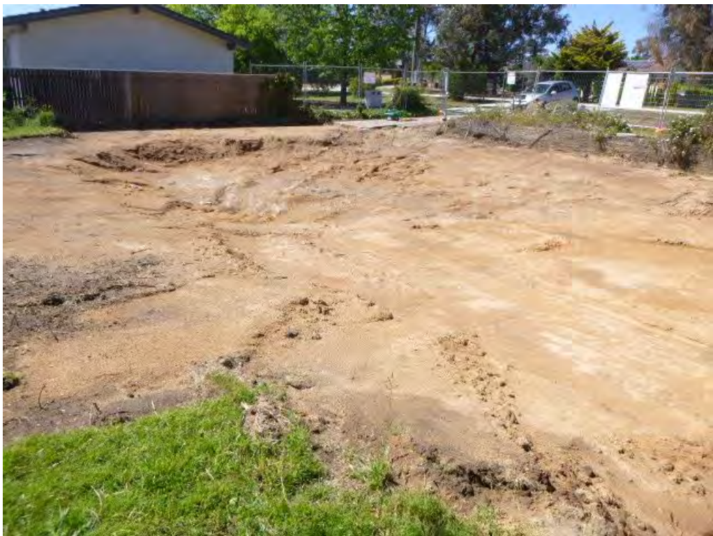
Figure 2 Site overview of demolition footprint.
