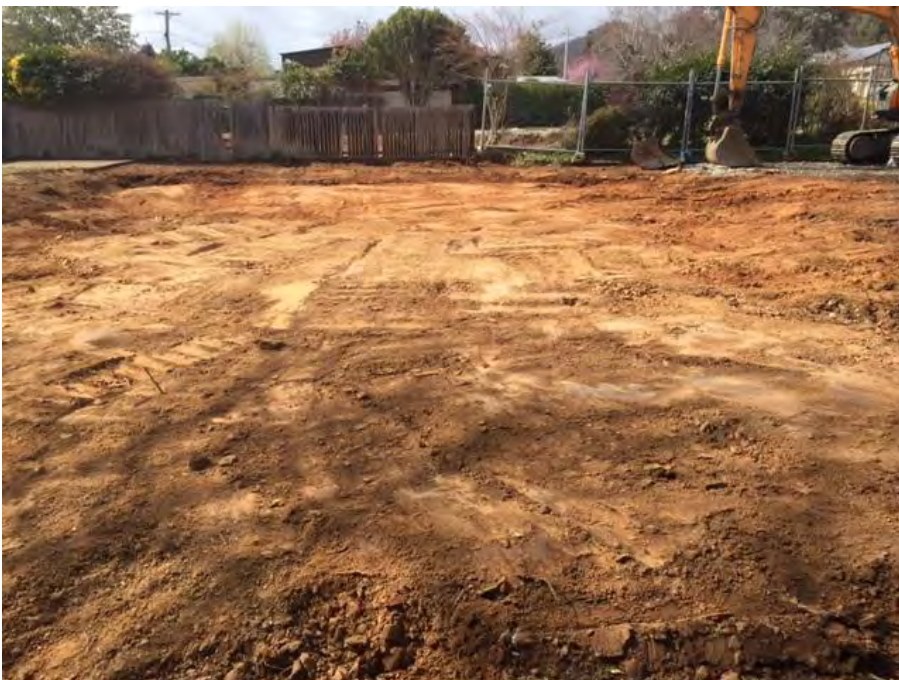
Photograph 2 – Dwelling footprint ground surfaces, taken from southwest side of the site
