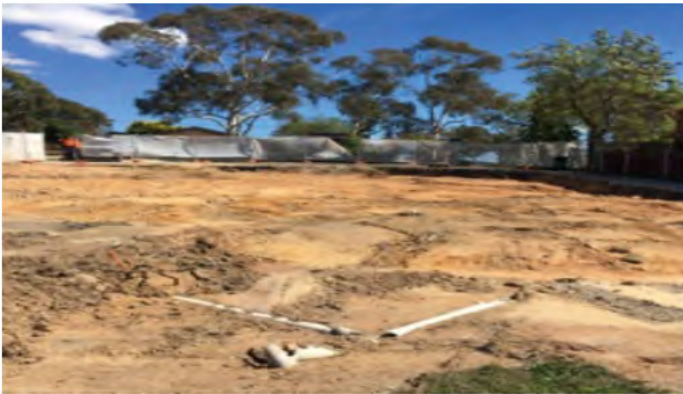
Cleared area of the demolition zone
