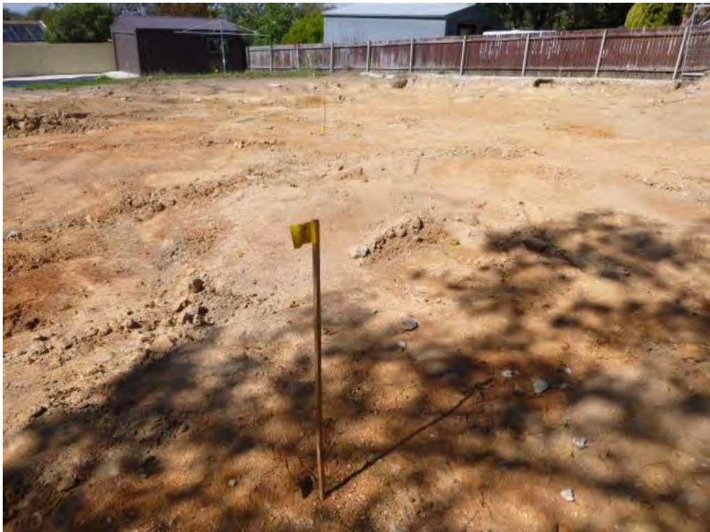
Figure 4 Soil validation sample location/s (from the left) view from the north-western boundary corner to the south-eastern boundary: S-11, S-10, S-03, S-05 and S-06.
