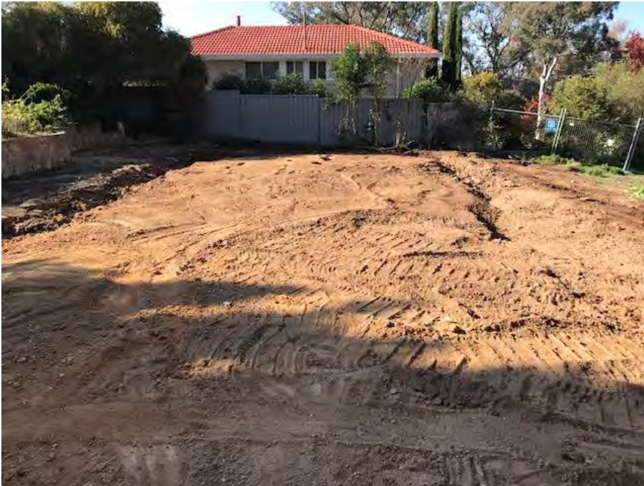
Photograph 3 – Dwelling footprint ground surfaces taken from West side of the site
