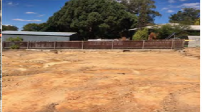
Cleared area of the demolition zone
