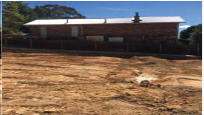
Cleared area of the demolition zone
