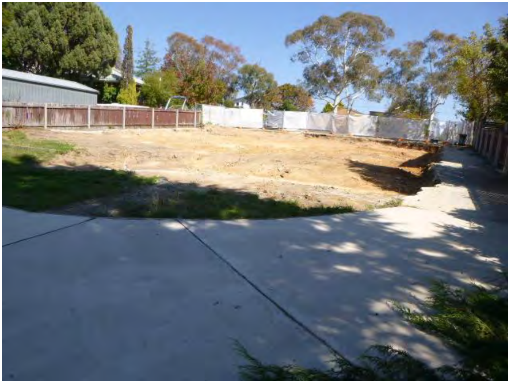
Figure 2 Site overview of demolition footprint.
