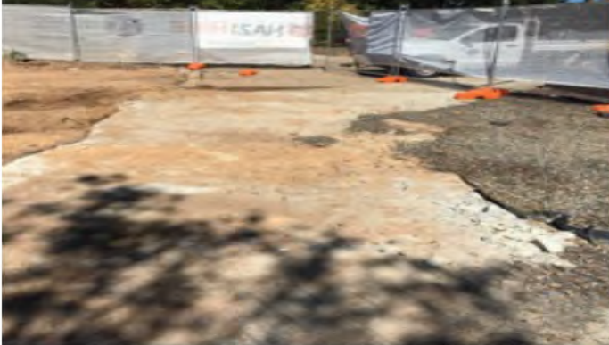
Driveway outside the demolition zone
