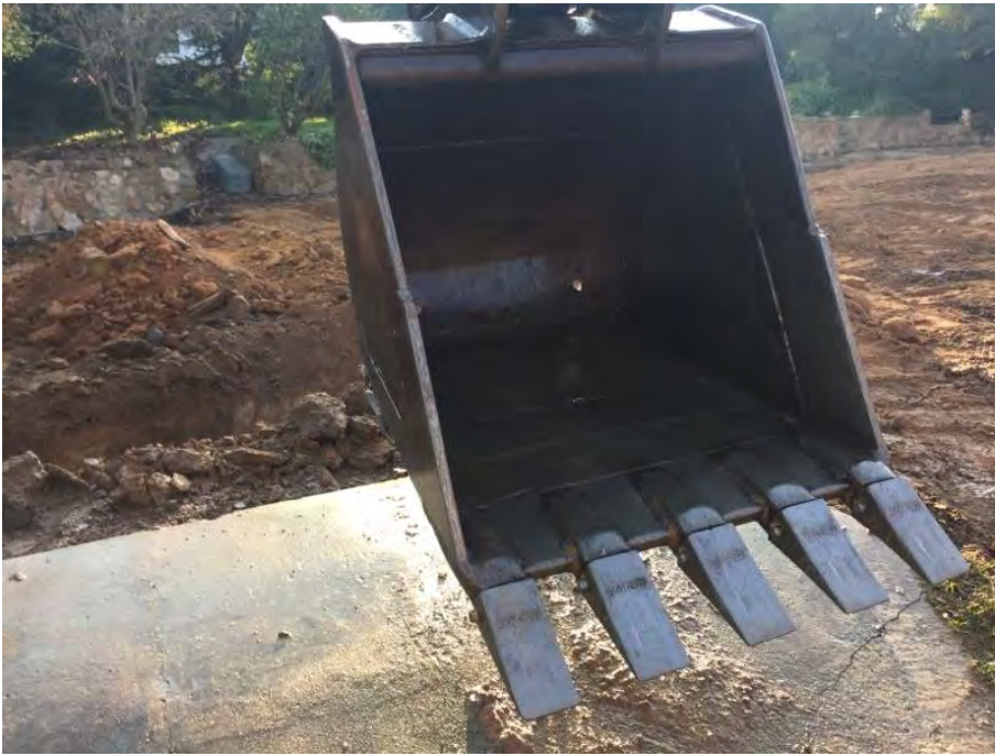
Photograph 7 – Excavator bucket after decontamination
