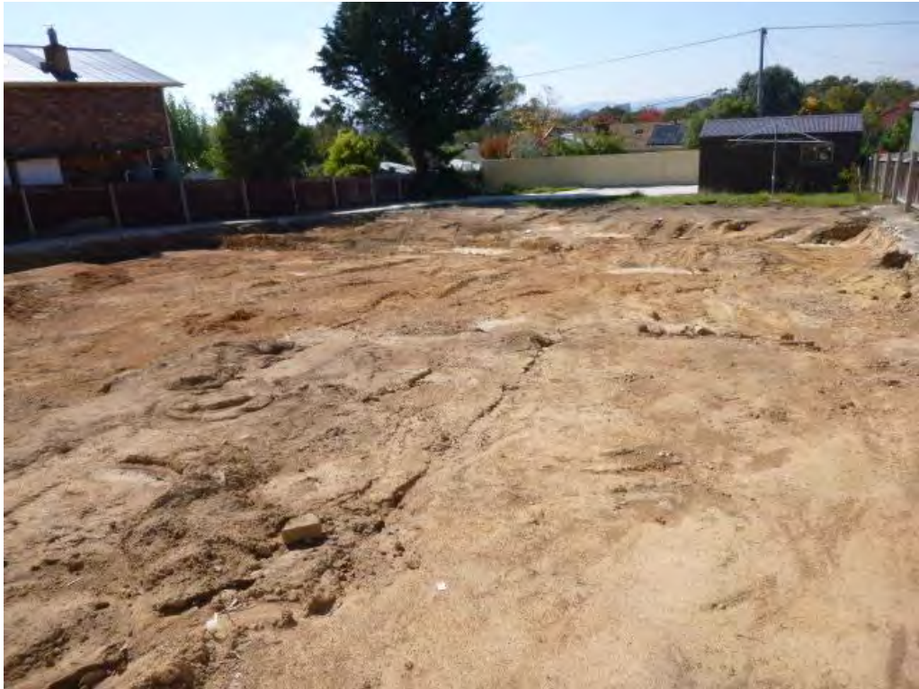
Figure 1 Site overview of demolition footprint.
