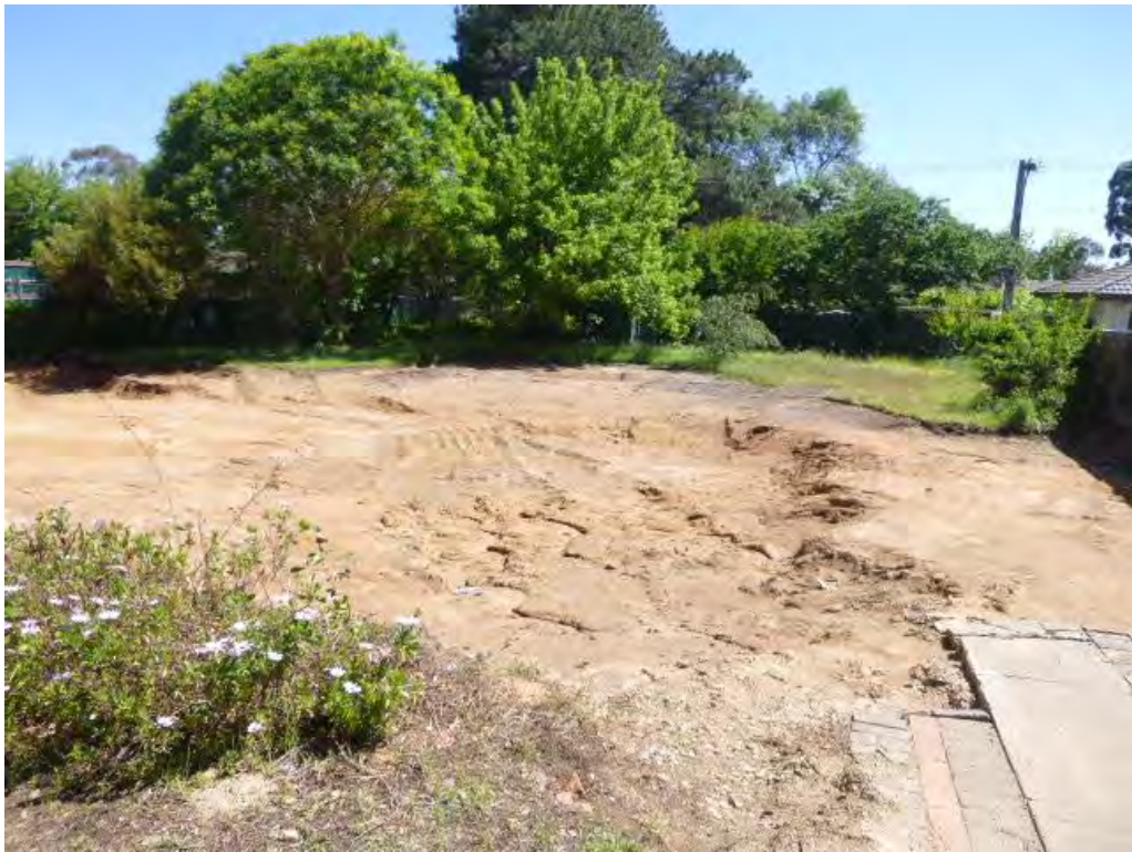
Figure 1 Site overview of demolition footprint.
