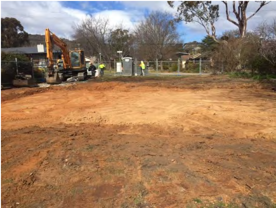
Photograph 3 – Dwelling footprint ground surfaces, taken from northwest side of the site
