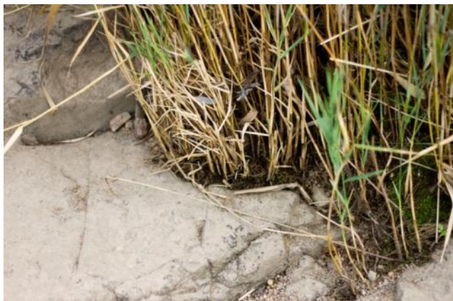
Figure 6 Built up sediment, weeds and native fauna may pose a threat to integrity of the grooves (ACT Heritage 2016).
