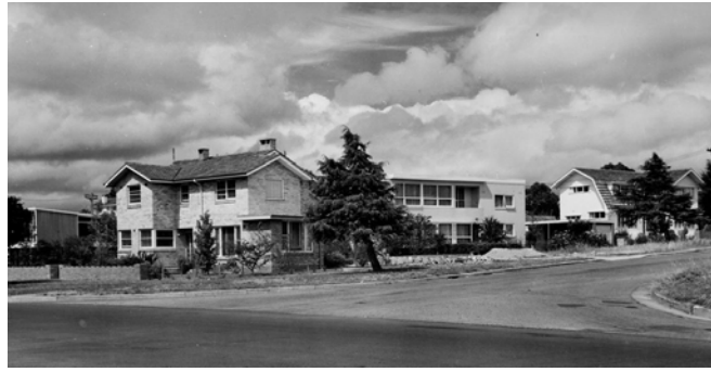
Later photo showing early extensions and alterations Image credit: Mr J. Gardner. EMA, 2016.
