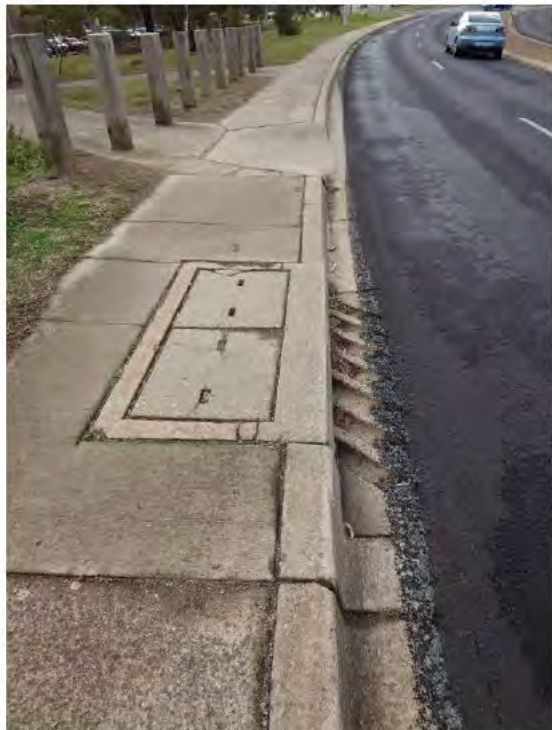
Figure 31 – Stormwater Sump on Redfern Street Looking East
