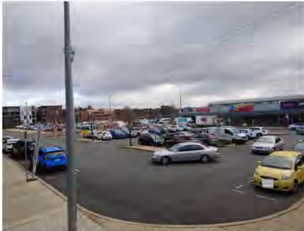
Figure 62 – TCCS Streetlights in Southern Car Park
