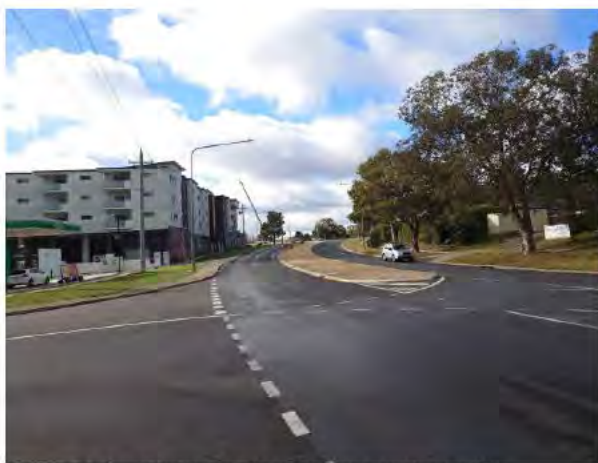
Figure 80 – Redfern Street Intersection with Bowman Street (east) Looking East
