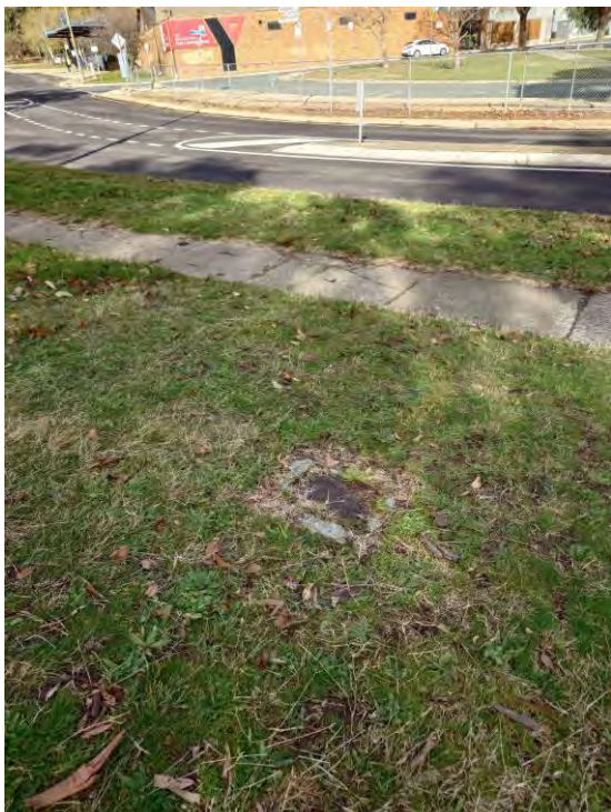
Figure 53 – Gas Marker Indicating Location of Branch into Site from Bowman Street (east)
