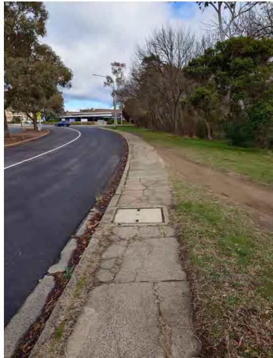
Figure 118 – Footpath in Northern Verge of Bowman Street (north) Looking South West
