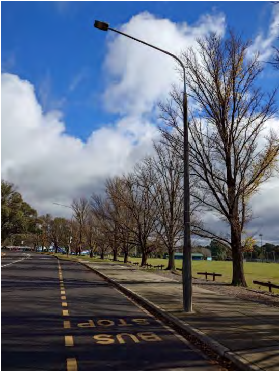
Figure 59 – TCCS Streetlight on Bowman Street (north)
