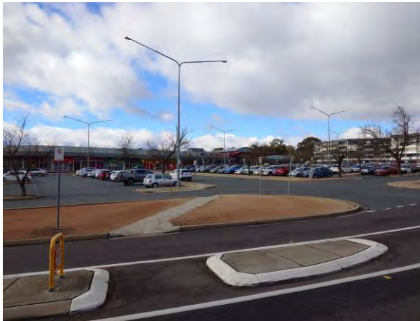
Figure 120 – Centre Island Refuge in Bowman Street (west) and Path to West Car Park
