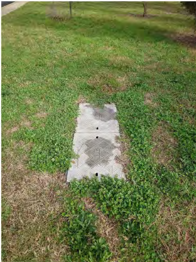
Figure 50 – TPG Pit in Northern Verge of Redfern Street South of Site
