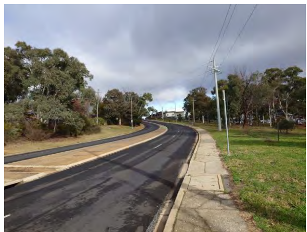
Figure 70 – Electrical Overhead Power Lines in Redfern Street Looking West
