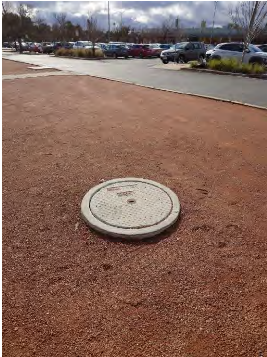
Figure 34 – Stormwater Manhole in Bowman Street (west) East Verge over DN600 Main
