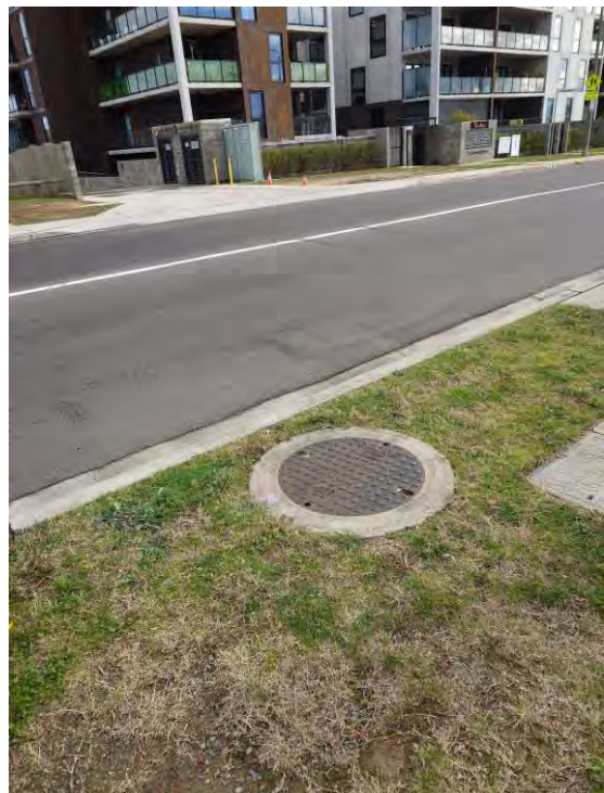
Figure 36 – Existing Stormwater Manhole South West of Site
