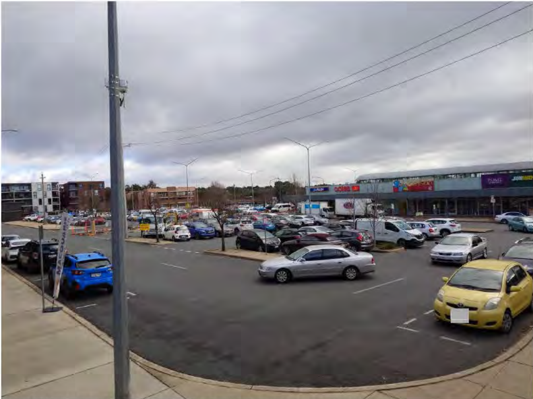
Figure 10 – General Site Photo Southern Car Park Looking North West
