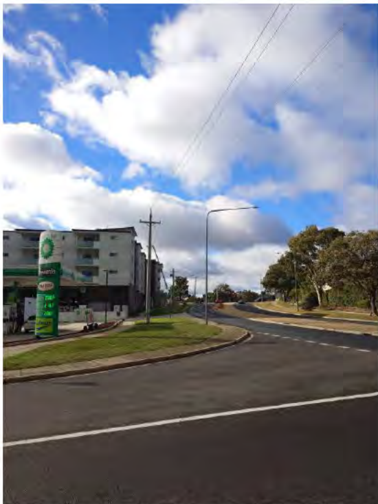
Figure 71 – Electrical Overhead Power Lines in Redfern Street Looking East
