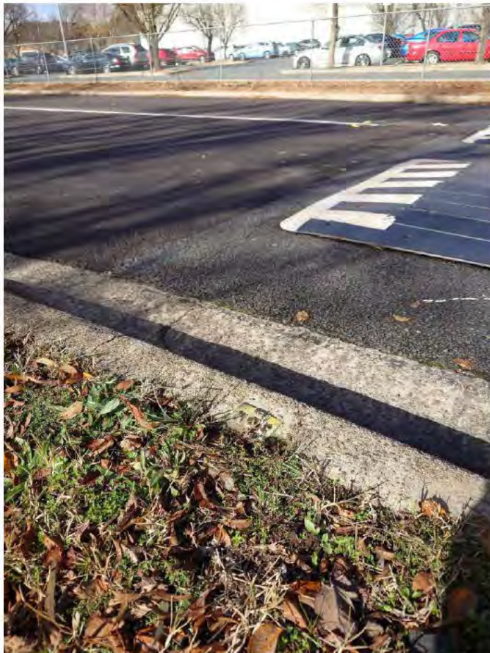
Figure 78 – Kerb Survey Marker KBM
