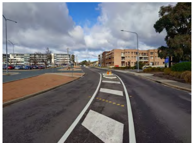
Figure 119 – Footpath in West Verge of Bowman Street (west) and Centre Island Refuge
