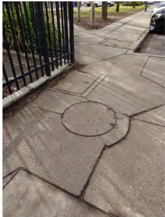
Figure 32 – Stormwater Sumps and Manhole in Redfern Street
