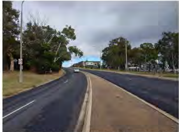
Figure 64 – TCCS Streetlights on Redfern Street Looking West
