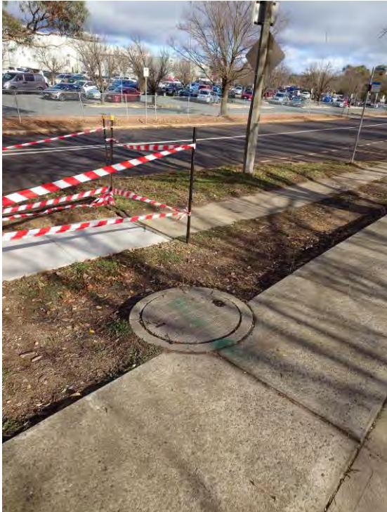
Figure 16 – Sewer Manhole in Bowman Street (north)
