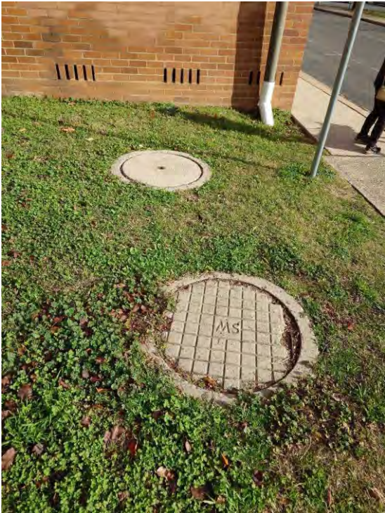
Figure 15 – Sewer Manhole (further) Near Block 10 Section 50
