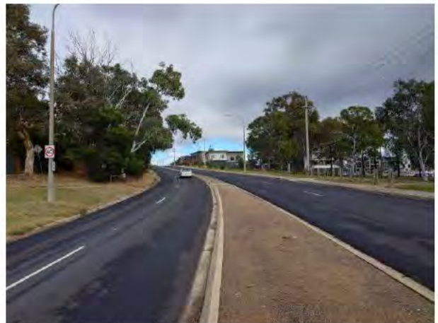
Figure 73 – Electrical Overhead Power Lines in Redfern Street Looking West
