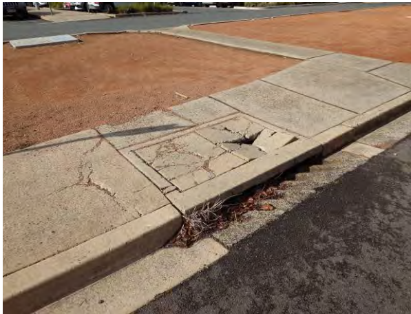
Figure 33 – Existing Stormwater Sump in East Verge of Bowman Street (west)
