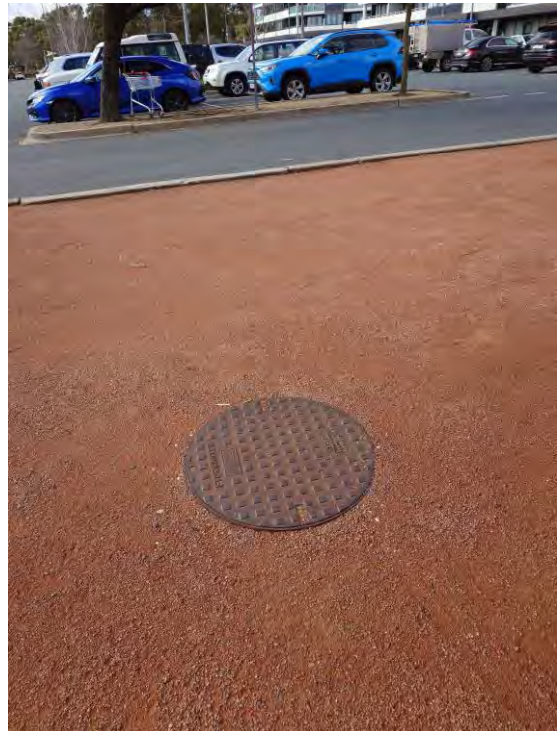
Figure 35 – Stormwater Manhole in Bowman Street (west) East Verge over DN675 Main
