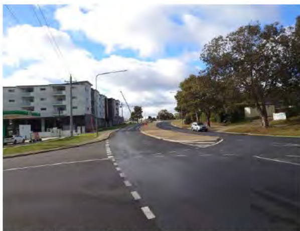
Figure 72 – Electrical Overhead Power Lines in Redfern Street Looking East
