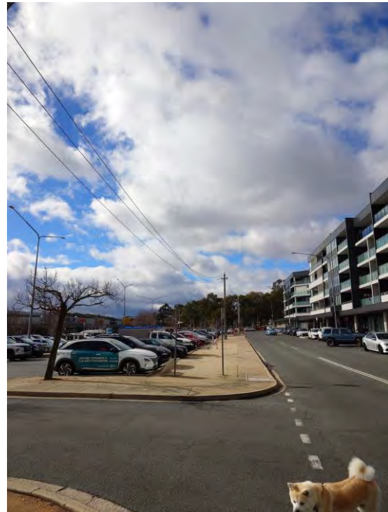
Figure 76 – Electrical Overhead Power Lines in Henshall Way Looking East
