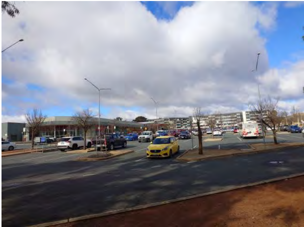
Figure 61 – TCCS Streetlight in West Car Park
