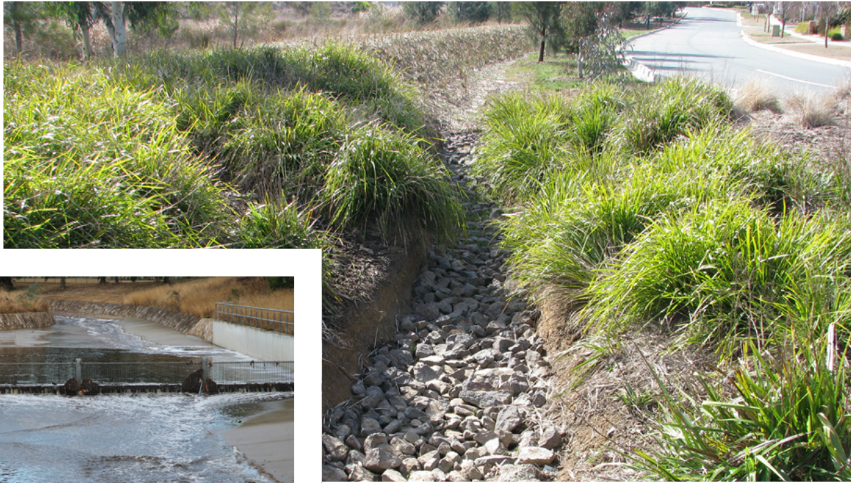
Rubble drain in Forde
