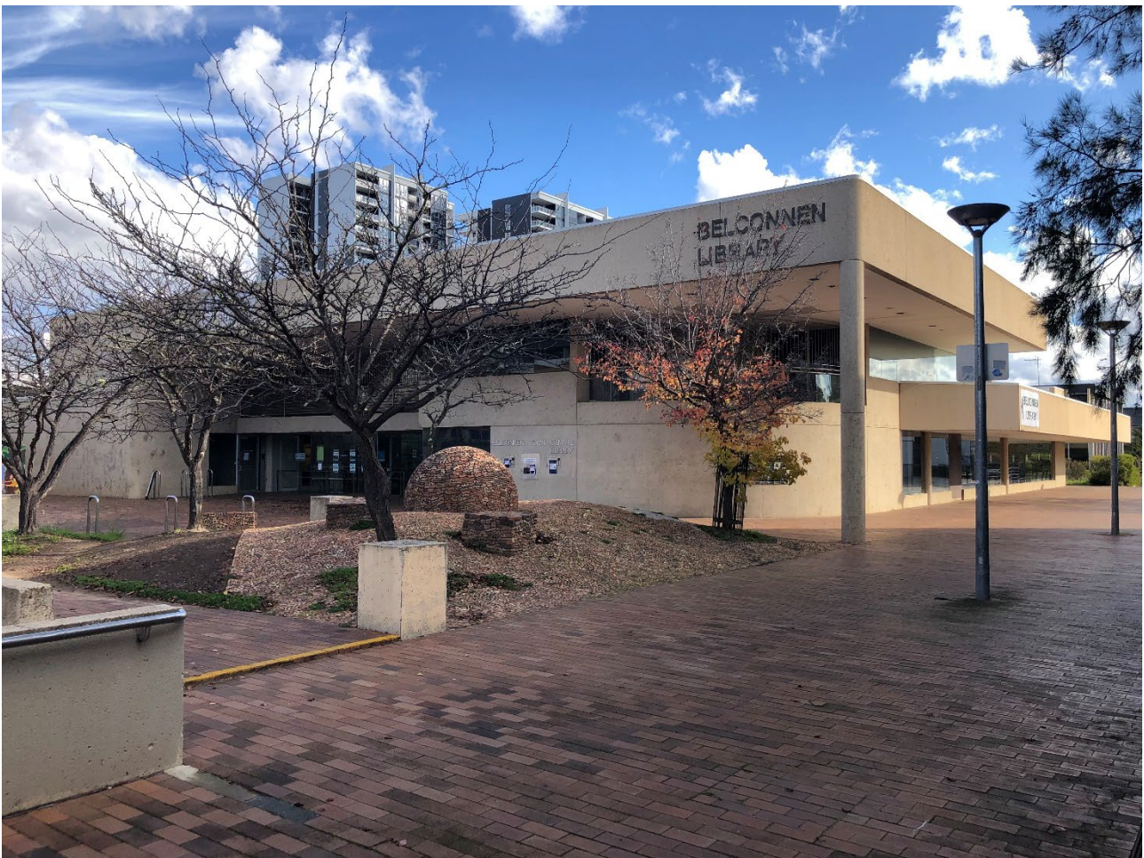
Figure 1 Belconnen Library from Chandler Street – view from Northeast corner (ACT Heritage, 2020)
