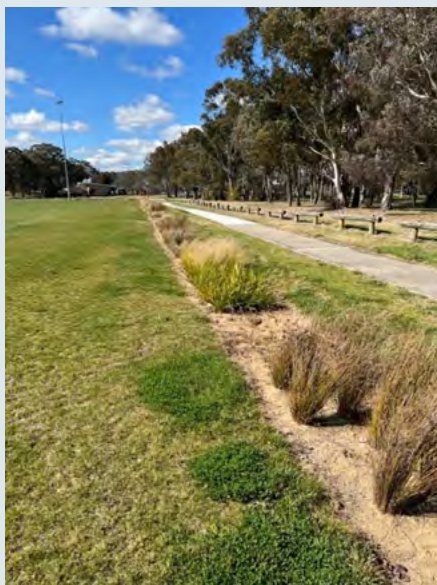
Bio retention swales at Kambah Photo credit: ACT Healthy Waterways, OoW
