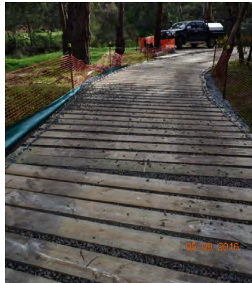
Figure 12: Rumble boards over crushed rock.
