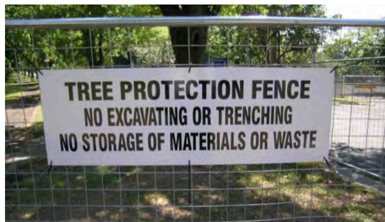
Figure 10: Example of a TPZ warning sign clearly displayed on TPZ fencing.
