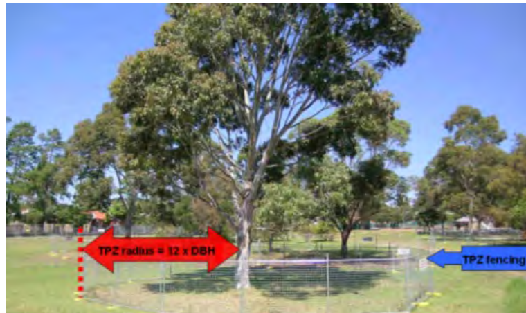
Figure 9: TPZ fencing is erected around retained trees prior to site works.
