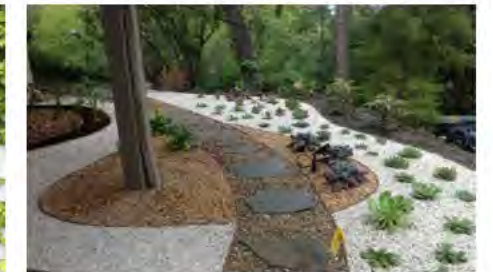
Car park drop-off area: bonded gravel garden
