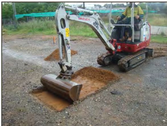
Figure 7. Mechanical excavation of the initial spits in TT1 (facing north-west).
