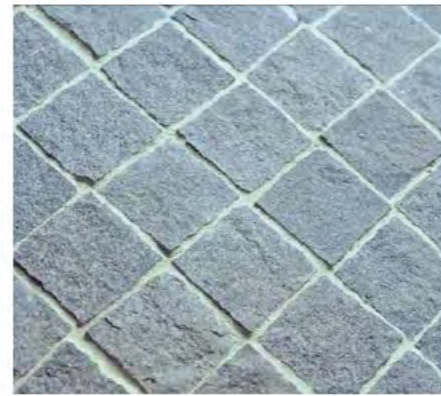
Paving Type 3: Cobble thresholds sets Granite
