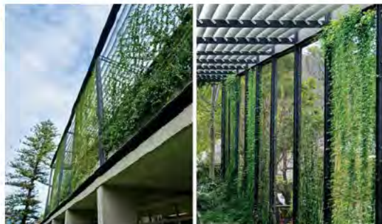
Mixed vines growing up tensile wire balcony to balcony to top of buildings
