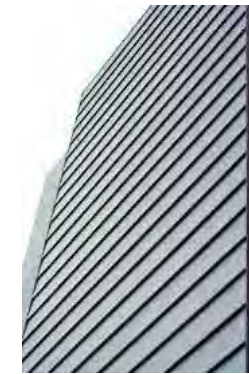
BALCONY CLADDING - TOWER
