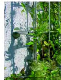
Cable trellis detail
