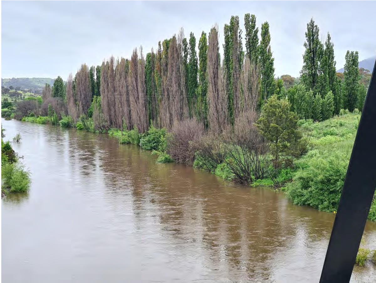
Figure 2 - Lombardy Poplars upstream of Tharwa bridge, 13 Nov 2021. Note the row of dead Poplar suckers, treated with herbicide and ready to be removed as part of this program.
