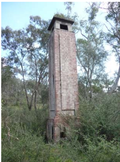
Ventilation shaft (feature # 36)
