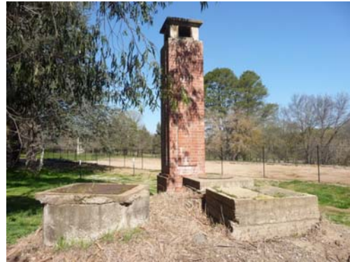
Ventilation shaft (feature # 22)
