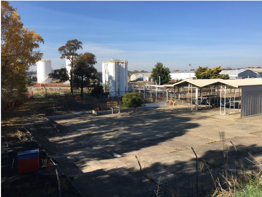
Figure 3 Residual fuel storage infrastructure onsite
