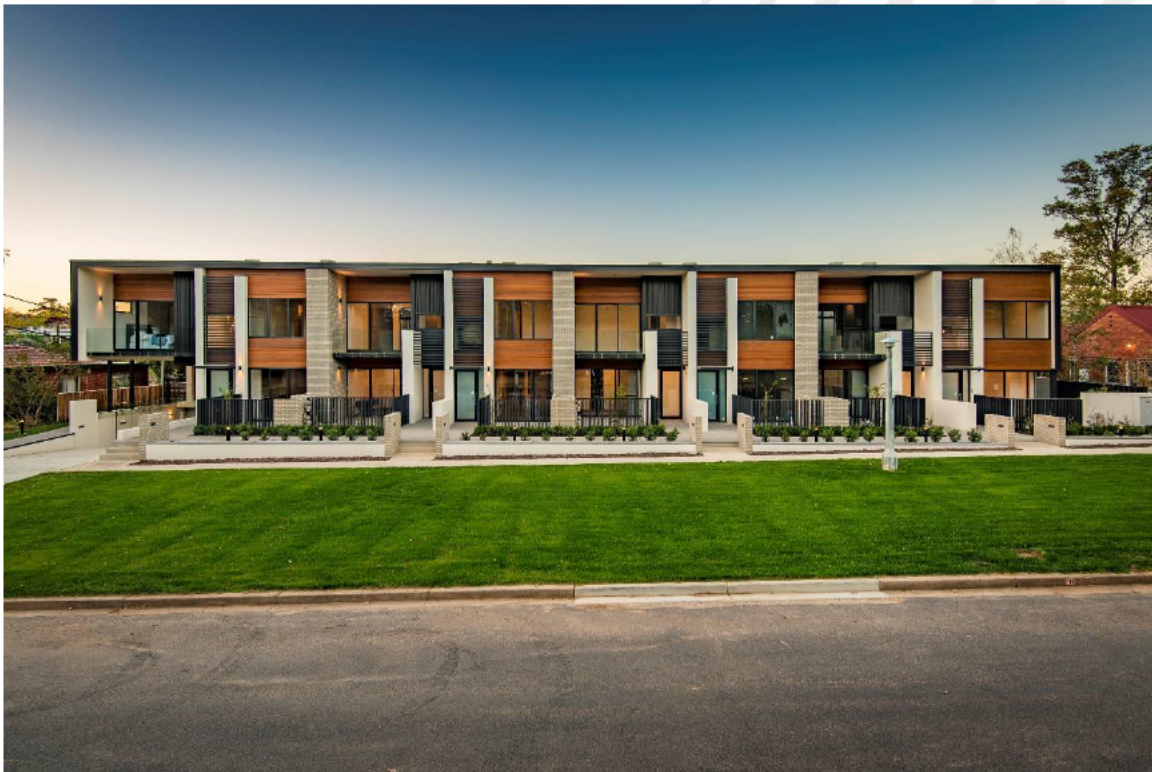
Existing 'Haig' development next door showing clear glass to the first-floor balconies
