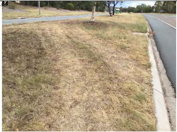
2 17Feb17 Southern Intersection Mortimer Lewis and Drakeford Drives. View across Drakeford Drive showing detail of beaten vehicle tracks.
