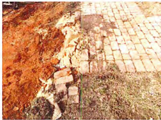
Paved area outside the demolition zone'
