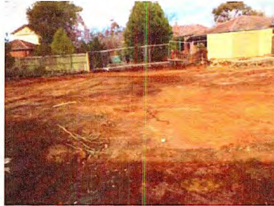
Cleared area of the demolition zone
