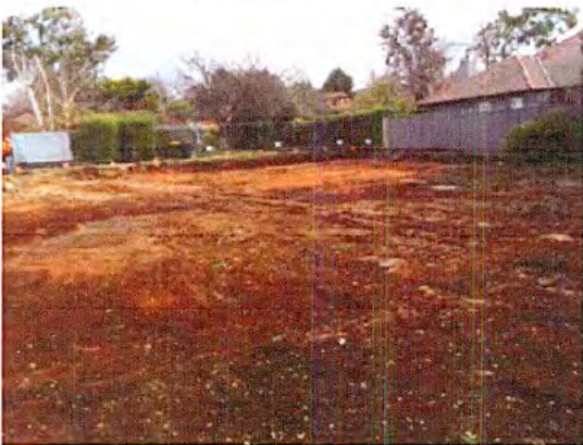
Cleared area of the demolition zone
