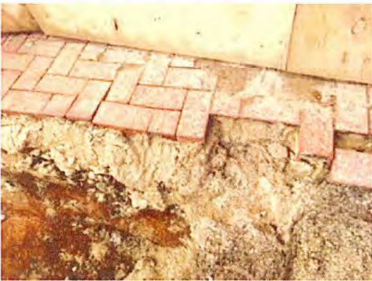
Paved area outside the demolition zone'
