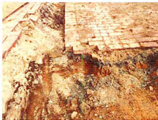
Driveway outside the demolition zone
