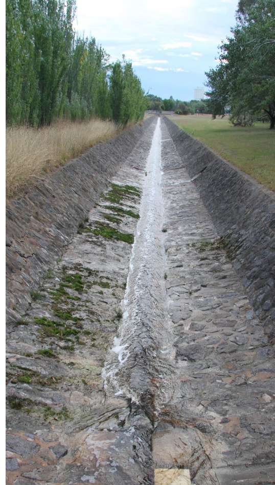
ARMOURED CHANNEL, WODEN
