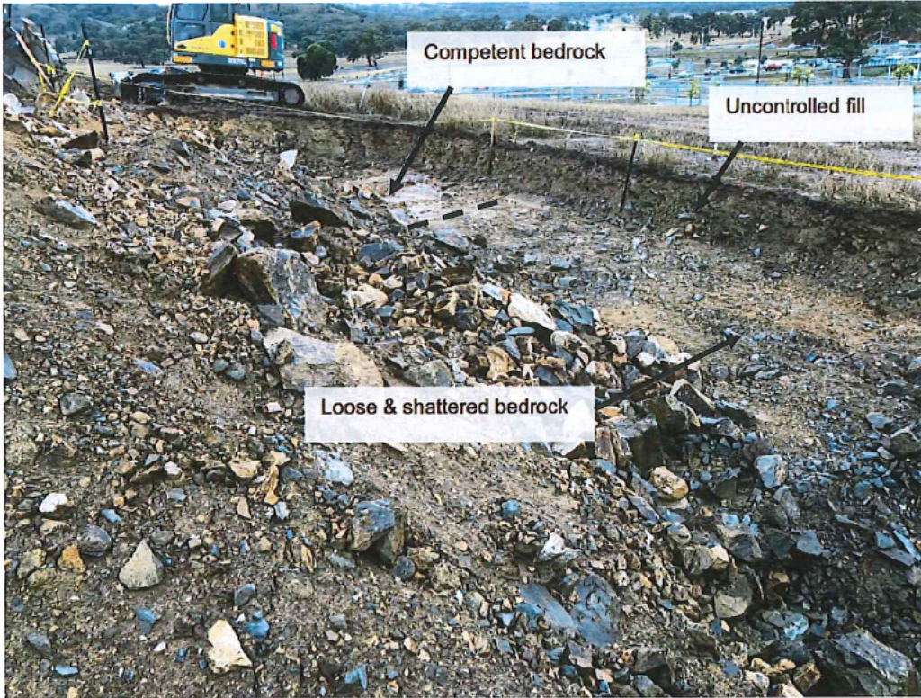
Photos 5 & 6 (above and below) – 26/2/2018 – View of the site cut in the western corner of the site, showing the loose, shattered bedrock extending to >2.8m depth. The transition between the competent bedrock, and loose, shattered bedrock can be seen in the rearground.
