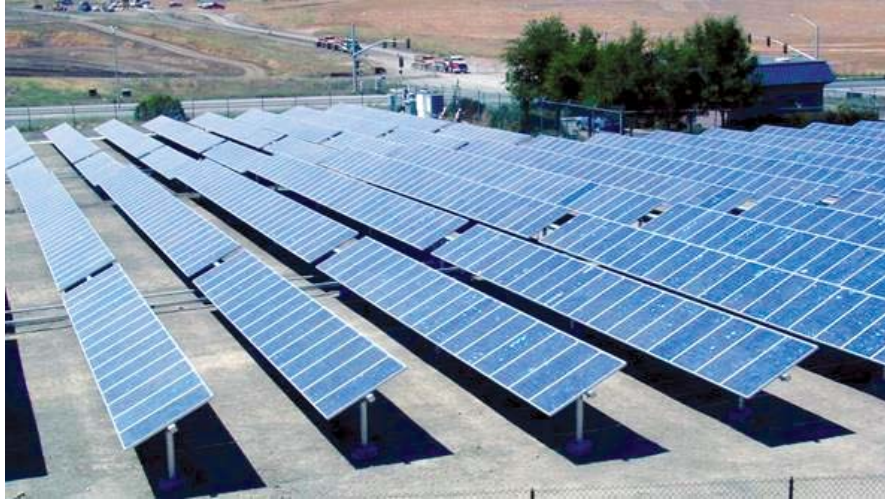
Figure 3-1: PV power plant, Domaine Carneros Winery, Napa, CA - 120 kW [Copyright: PowerLight Corporation]
