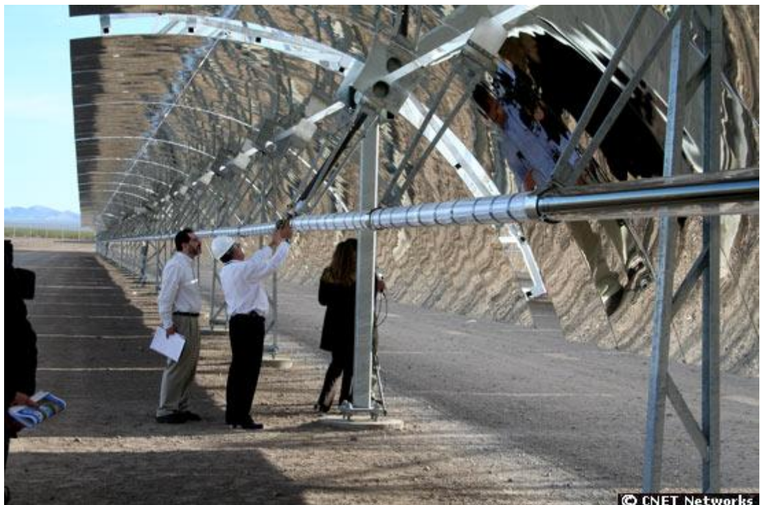
Figure 5-4: Partially stowed trough reflector
