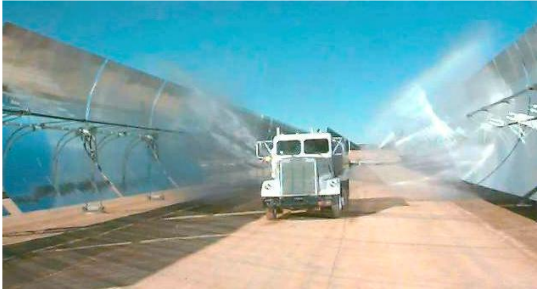
Figure 5-5: Trough reflector cleaning at SEGS
