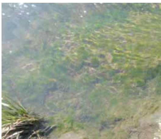
Spring tufts of conspicuous green algae on a concrete culvert. Poor riparian vegetation encourages compensatory growth of filamentous algae.
