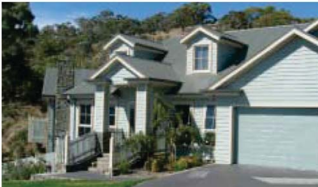
Broken roof planes combinations of materials provide visual interest
