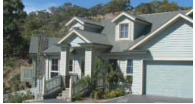
Broken roof planes combinations of materials provide visual interest
